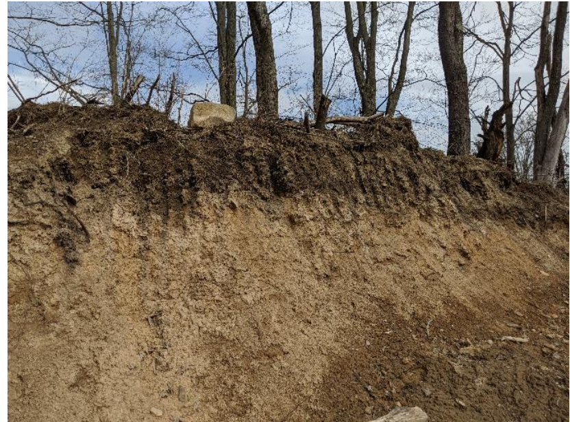
Photo 49. Edge of excavation and trees at top of ridge, facing east. 3/16/2020.
