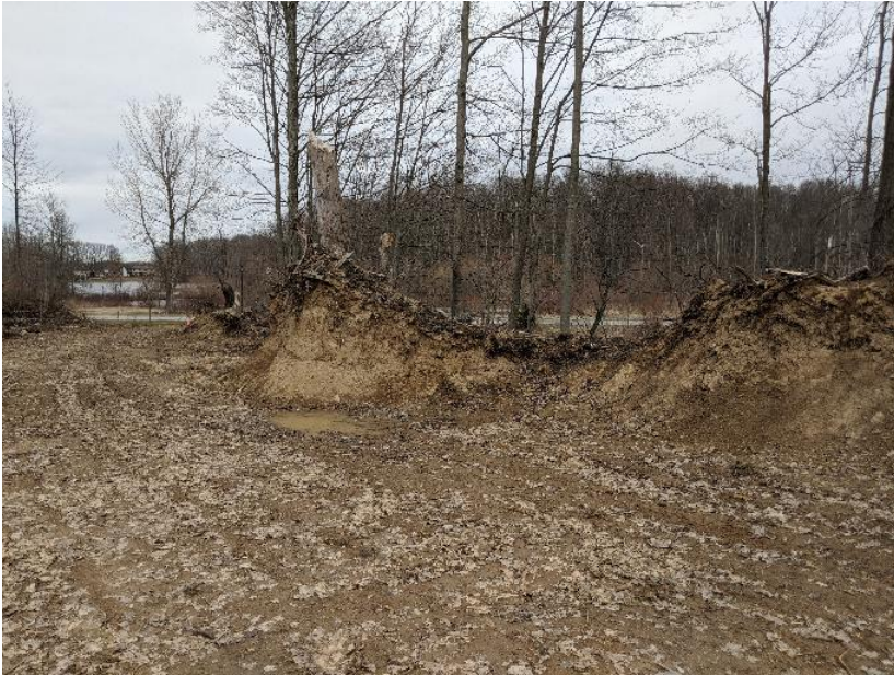
Photo 48. Facing northeast, showing excavation. 3/16/2020.
