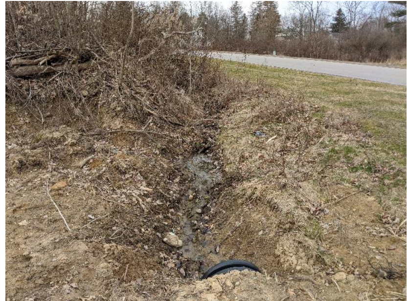
Photo 37. Facing west along roadside ditch. 3/16/2020.
