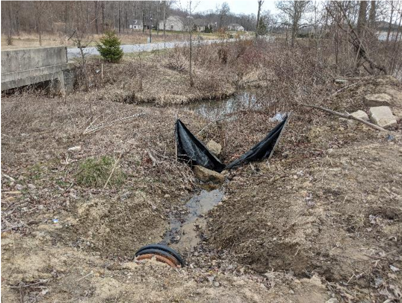
Photo 38. Facing east toward Burgess Run. 3/16/2020.
