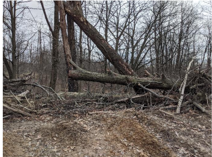
Photo 43. Facing south toward end of disturbed earth area. 3/16/2020.
