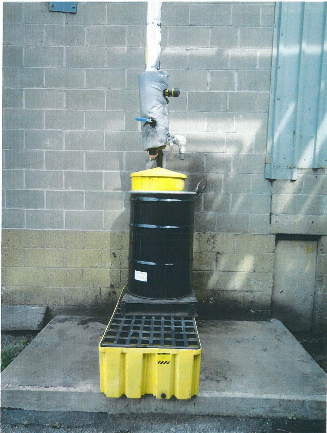
Photo #30: Closed 55-gallon container outside Sanyo Building #3000 (Aclube Unit), labeled as hazardous waste "Aclube Condensate", "D001, U162". Not dated. Label was not visible, facing wall. Facility manages container as a Satellite Accumulation Area.
