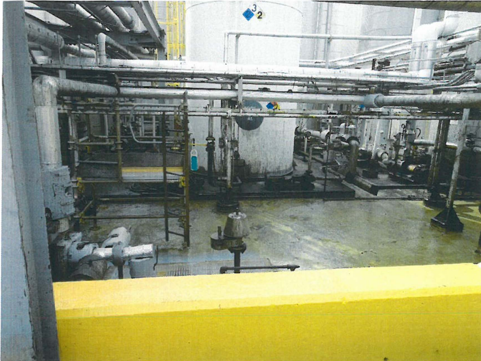
Photo #29: Overview of area from Photo #29. Sump from Photo #29 is in the foreground, just beyond the yellow wall.
