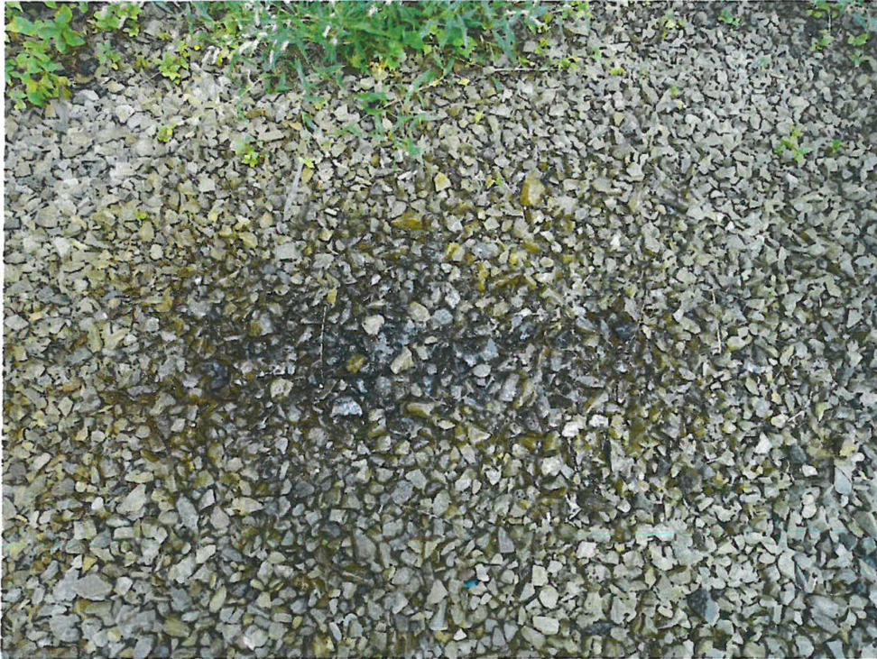
Photo #1: Stones adhering together, covered in material that leaked from overhead piping, outside the 160 Battery containment, specifically, behind tank 161. Area approximately 2 feet in diameter.
