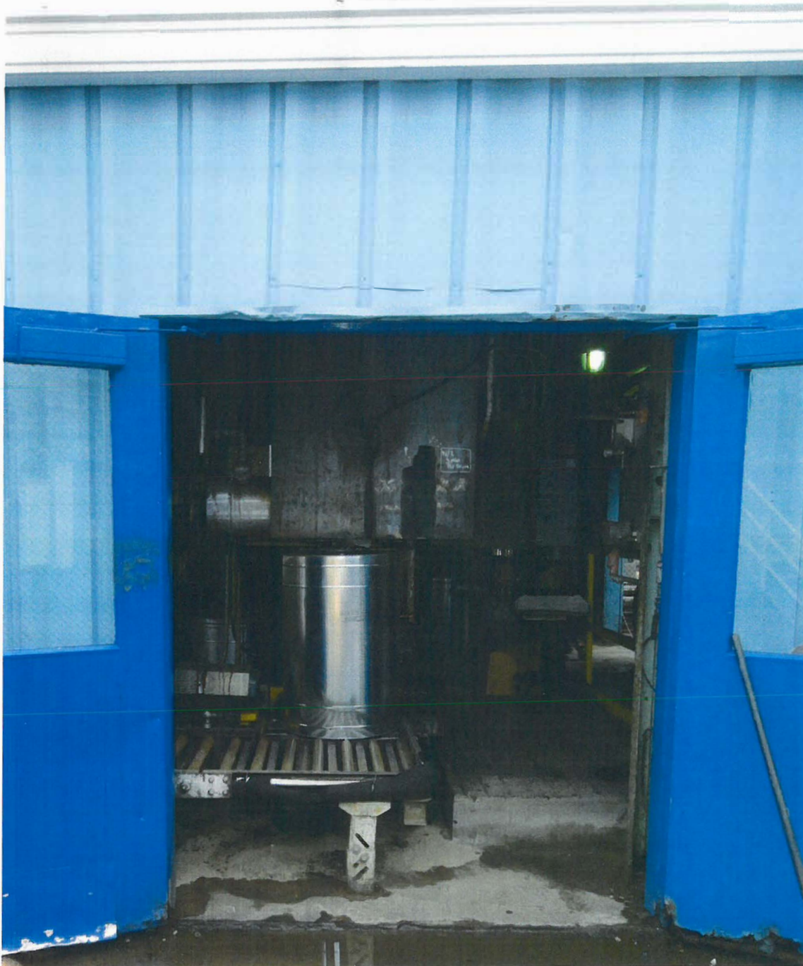
Photo #8: Drumming Station at the LTC-1 Unit, with spilled material on the floor, migrating out of the building.
