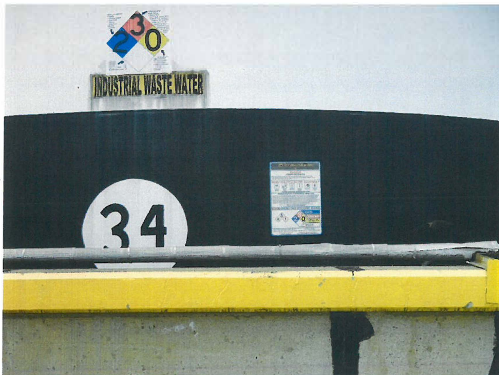
Photo #19: Close-up of markings on Tank 34, located south of, and adjacent to , the Battery 20 Dike. Tank 34 labeled as "Industrial Wastewater".
