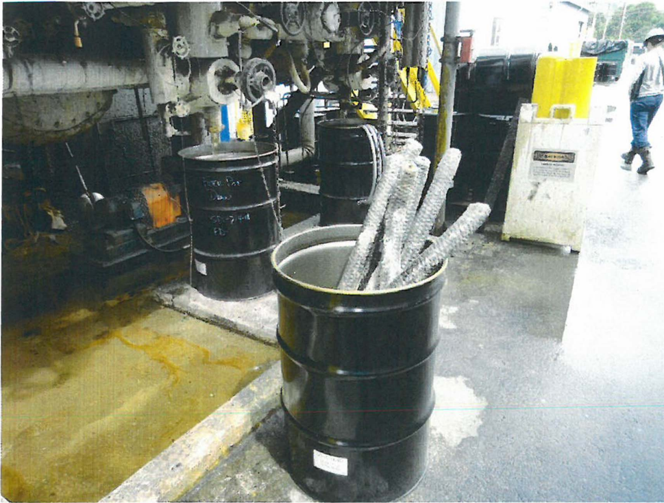
Photo #11: (3) open 55-gallon scrap resin containers in the Filter Pot Drain Drum Area. Container in foreground with waste filters. Container back left labeled “Filter Pot Drain”, and marked with a start date (SD) of 7-4-18.
