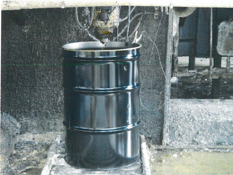
Photo #10: Unlabeled, open 55-gallon "scrap resin" collection container, in the Filter Pot Drain Drum Area. Container is connected to a ground wire.
