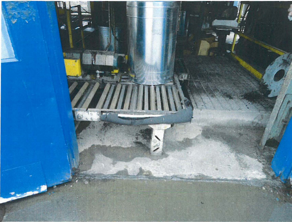
Photo #9: Close-up of spilled material from Photo #7. Spilled material migrating out of the building, onto the facility road.
