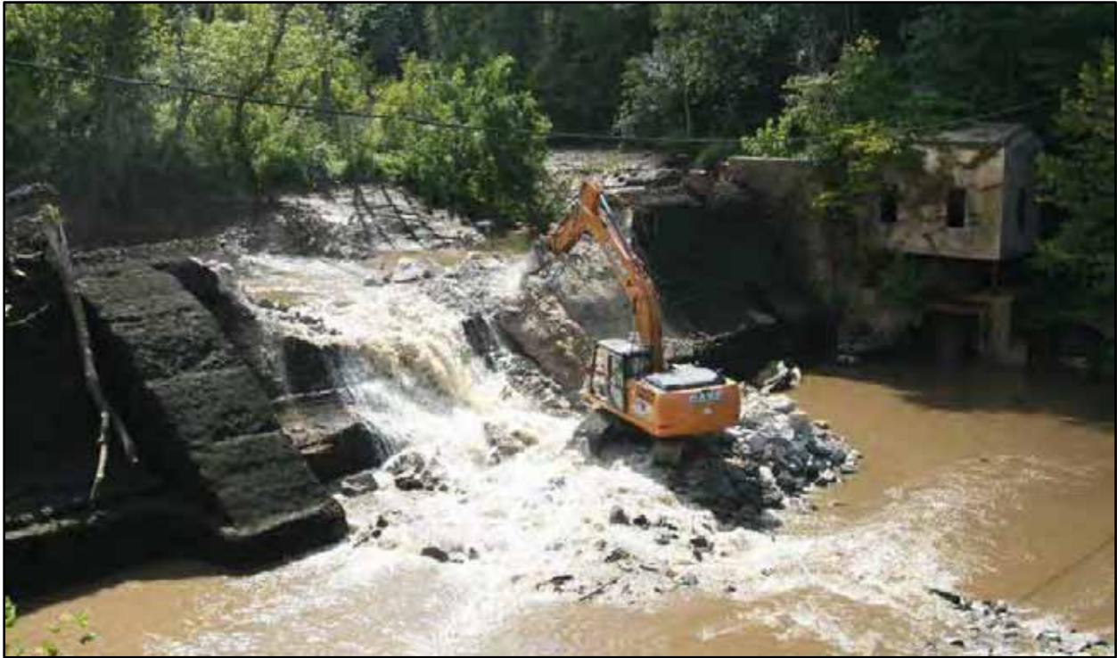
12. Progress of breaching activities after one day of work, view southeast (8/30/16) (credit FORVA)
