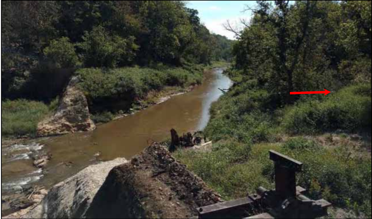
37. Re-established river channel and vegetated floodplain upstream of breach. Arrow depicts pool elevation (9/26/17)
