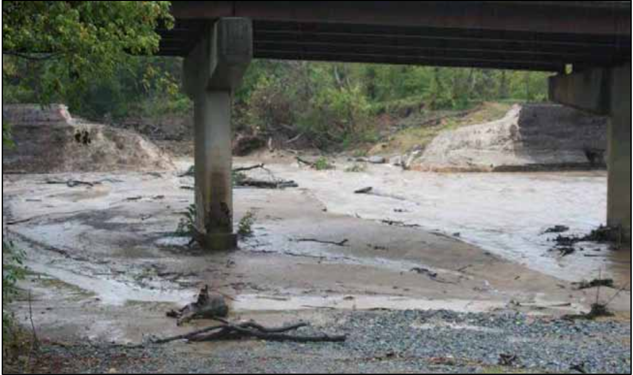
25. Floodplain deposition in downstream scour area during high flow event, view southeast (11/9/16) (credit FORVA)
