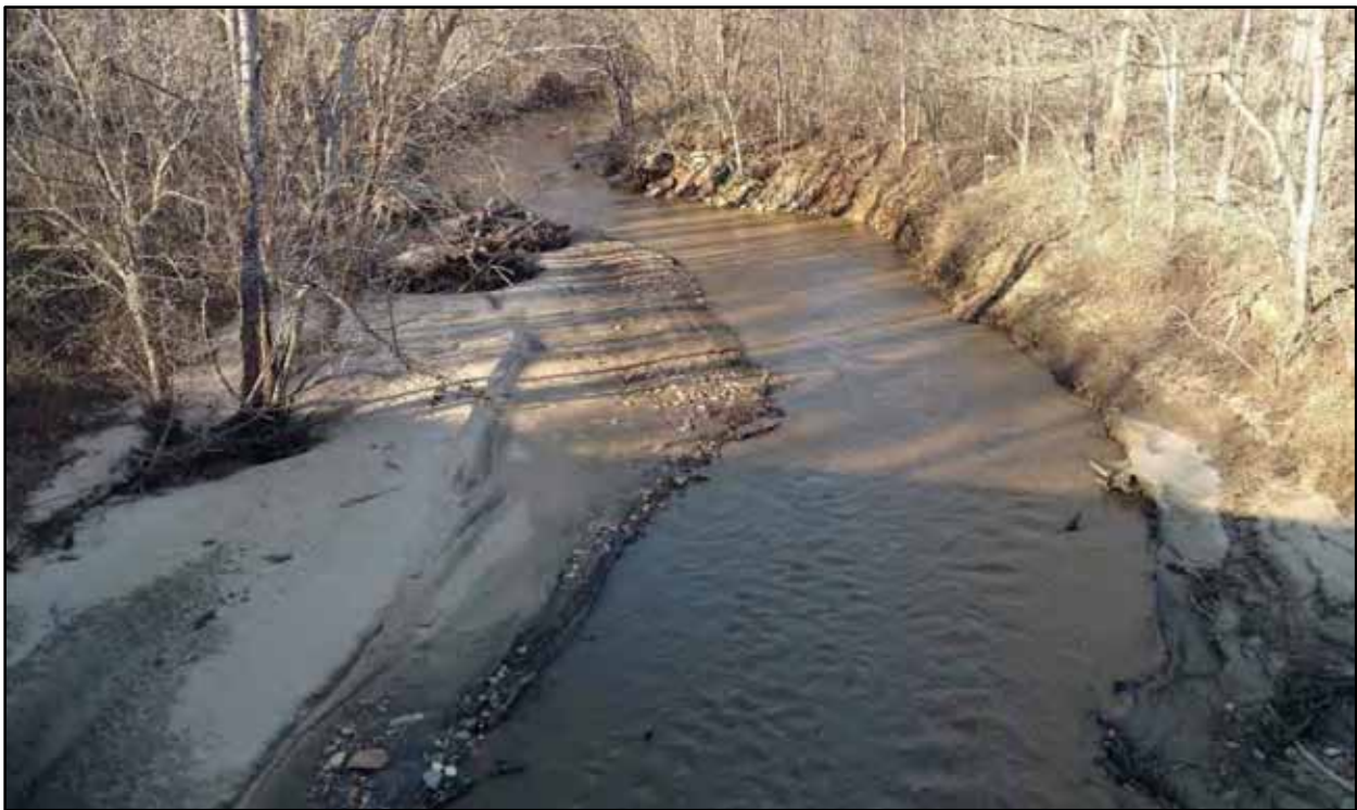
28. Narrowing of channel and restoration of meanders downstream below Route 712 Bridge (2/2/17)
