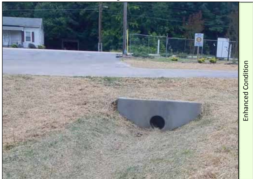
Picture 8: New headwall added to existing culvert.
