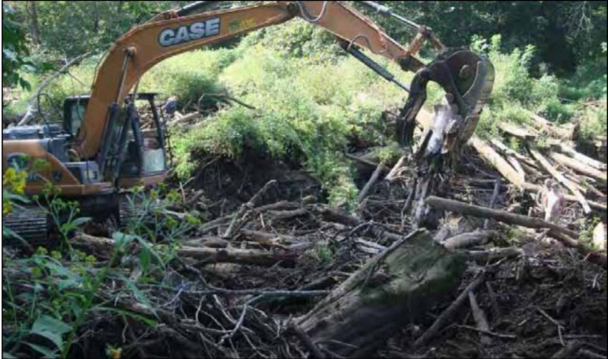
15. Removal of woody debris above Power Dam (9/9/16)
