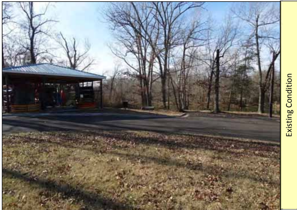
Picture 17: Existing storage building and proposed area for restroom.
