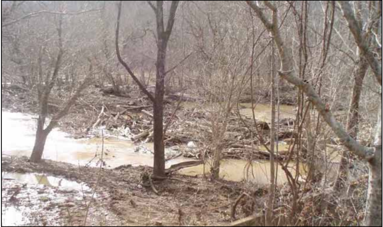
3. Woody debris upstream of Power Dam blocking river channel pre-breach, causing adjacent flooding (1/26/06)
