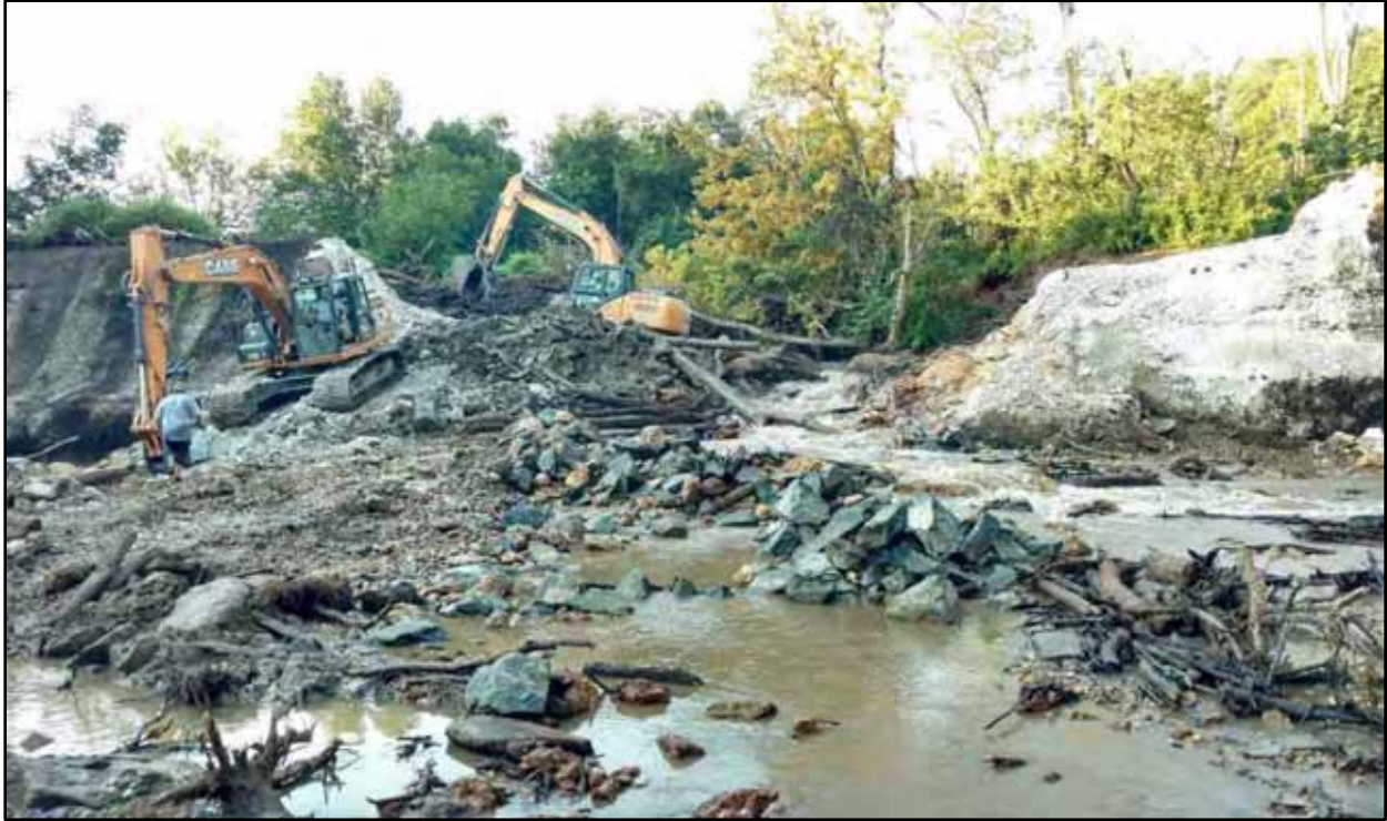
13. Woody debris removal behind Power Dam breach begins, view east (9/7/16)
