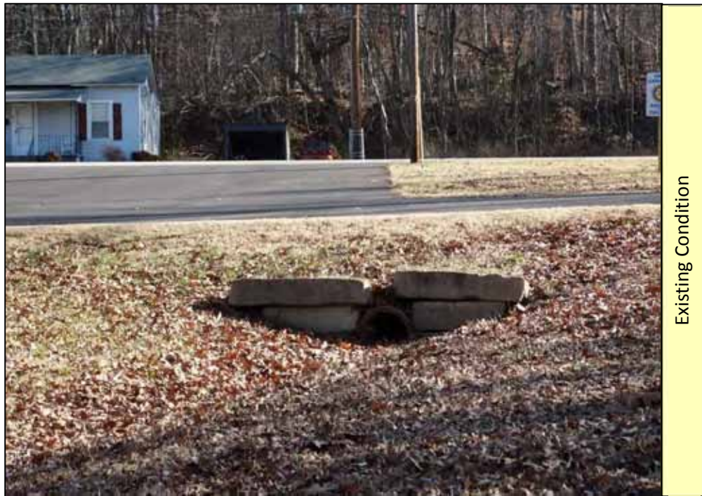
Picture 7: Existing culvert to receive new headwall.
