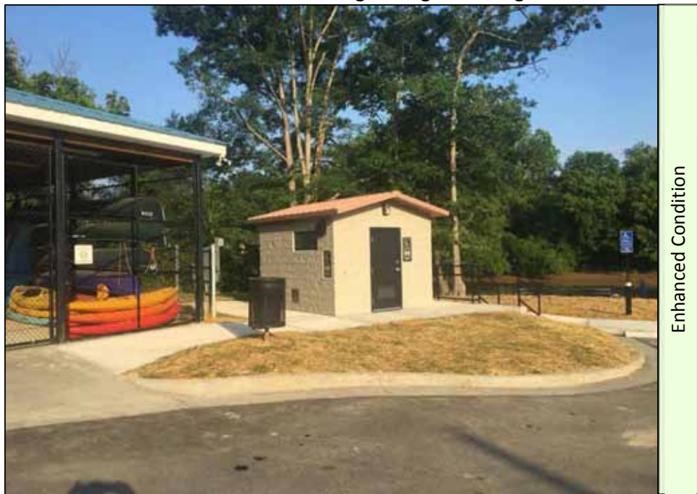
Picture 18: New restroom next to the existing storage building.
