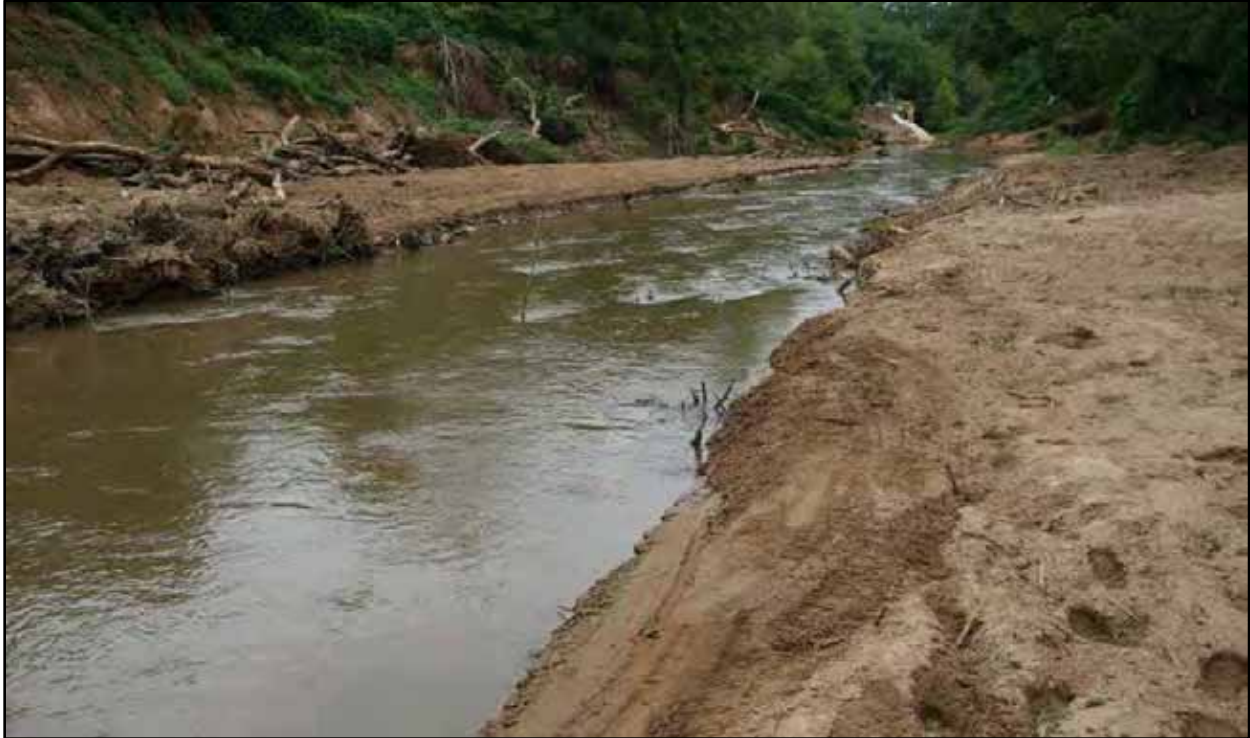
31. Floodplain bench and channel post fallen tree removal (breach in background) (8/2/17) (credit FORVA)
