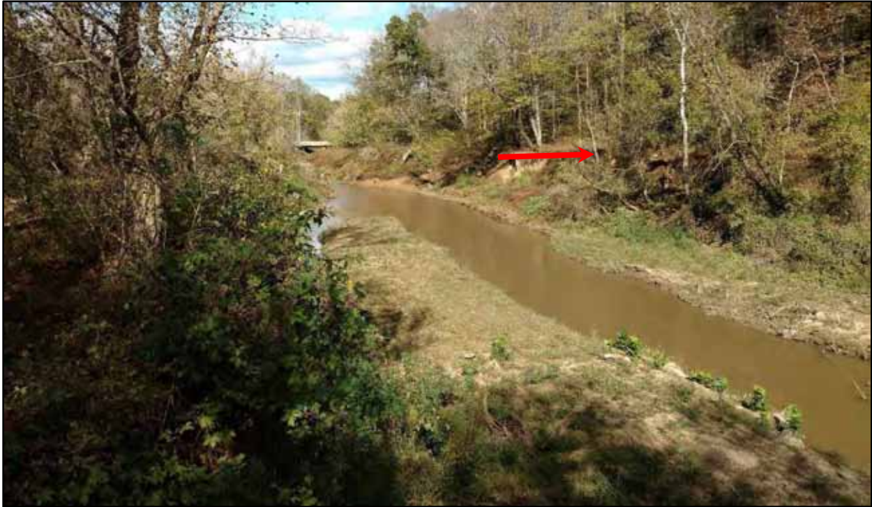
38. River channel and floodplain approximately 580 feet upstream of breach. Arrow depicts pool elevation (10/25/17)
