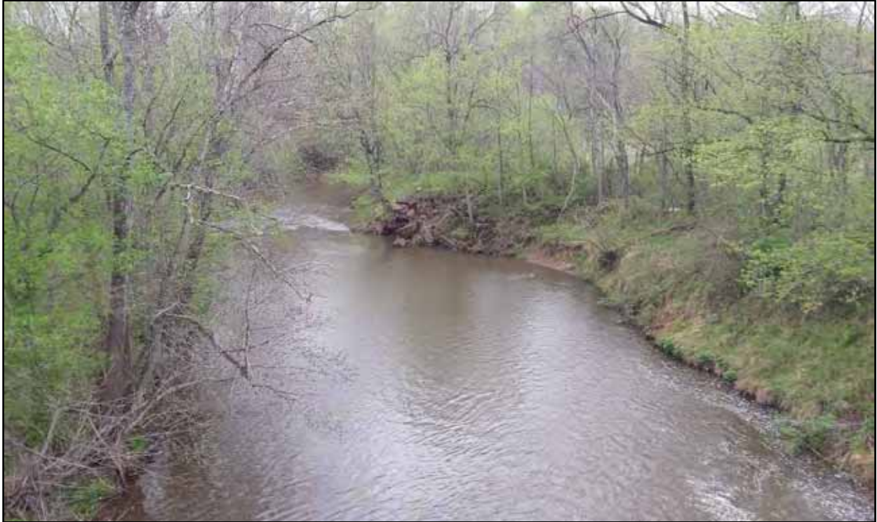
7. View north, downstream of Power Dam depicting over-widened, sediment starved channel (4/16/15)
