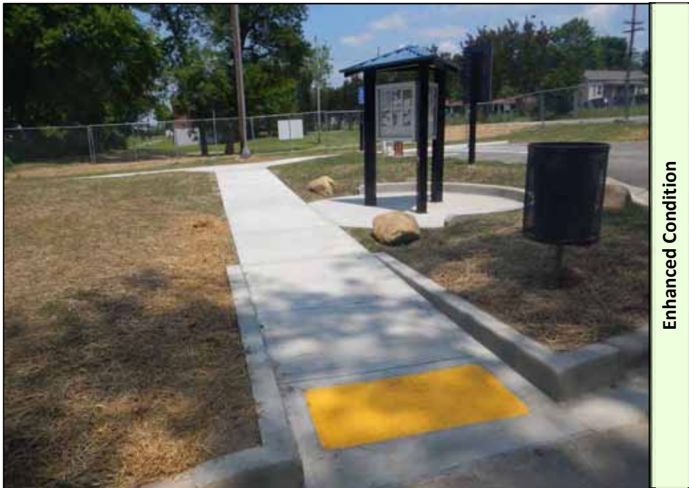
Picture 4: Added new accessible sidewalk leading to the kiosk and courtesy dock.
