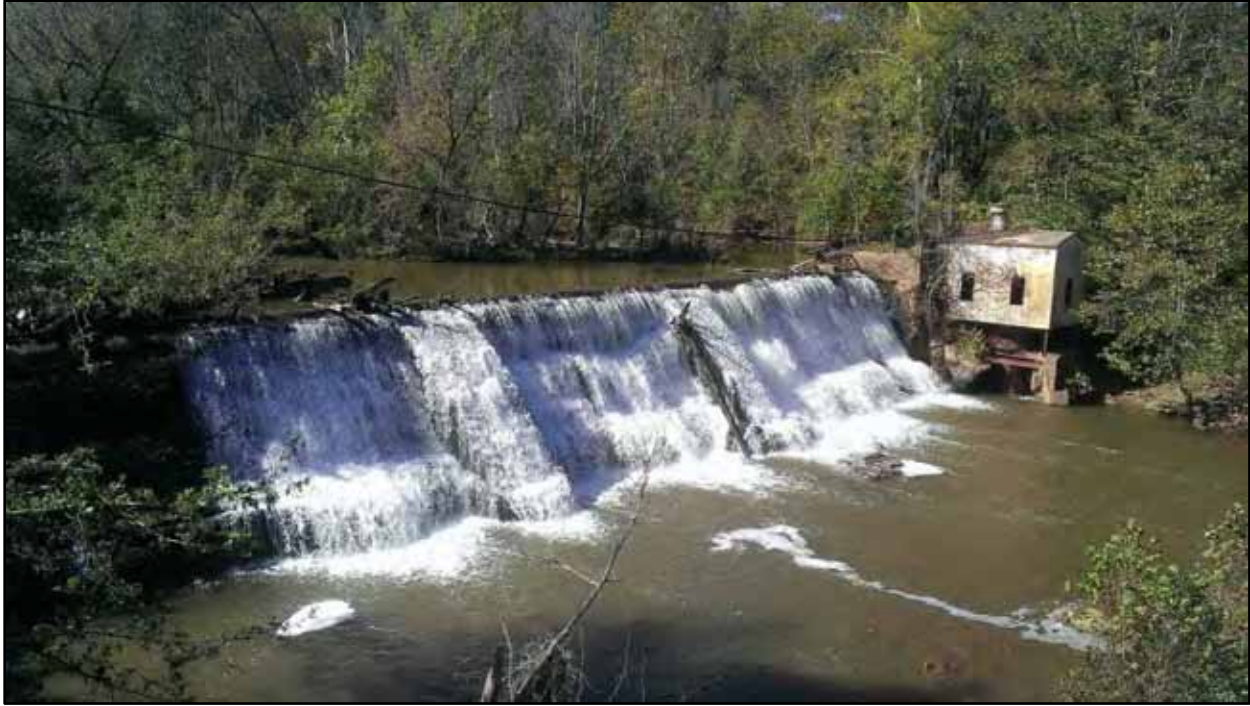
1. Power Dam pre-removal view southwest from Route 7124 Bridge (10/8/15)
