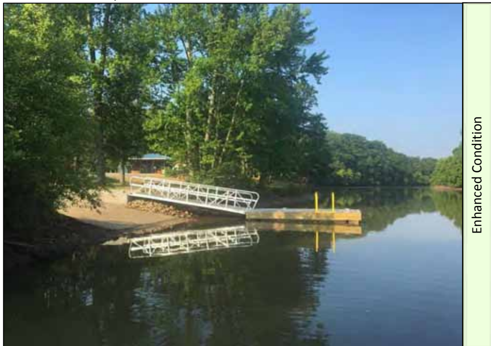
Picture 12: New courtesy dock.
