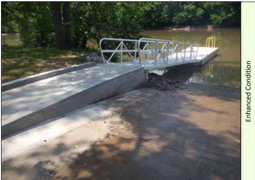
Picture 10: New accessible courtesy dock and connecting sidewalk.
