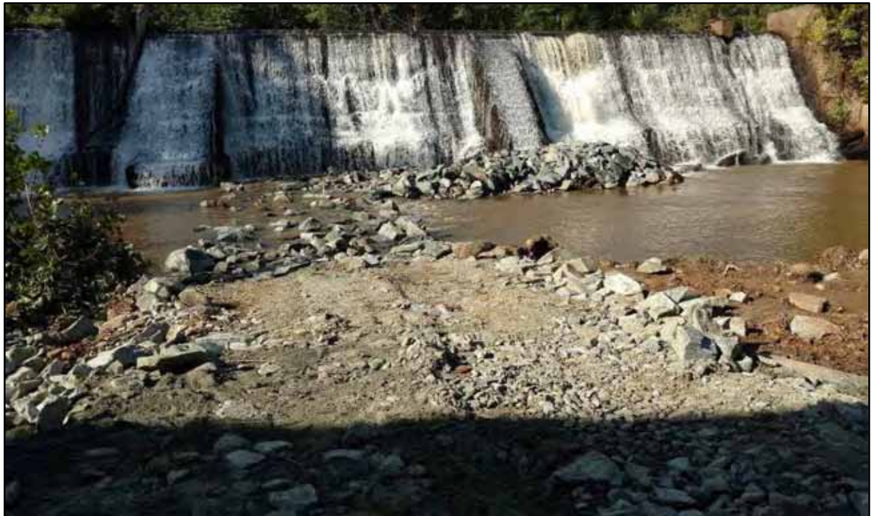
10. Construction access causeway in place prior to removal, view north (8/25/16)
