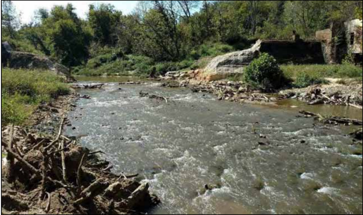
35. Riffle re-established in former scour hole below Power Dam breach (9/26/17)
