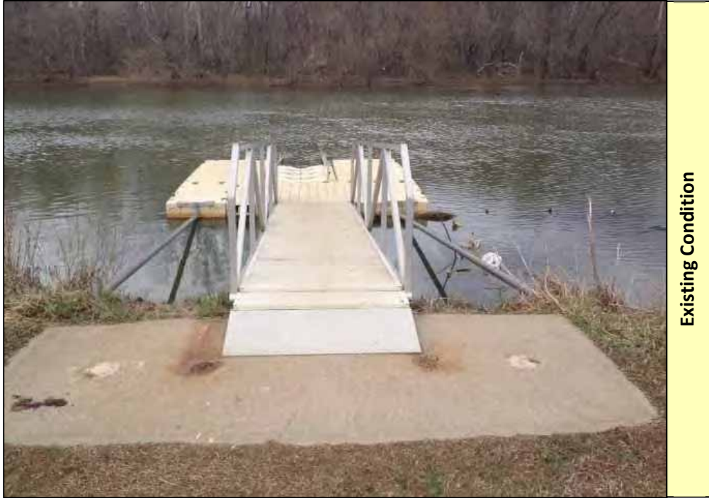
Picture 1: Existing floating dock and canoe launch. No enhancements planned.
