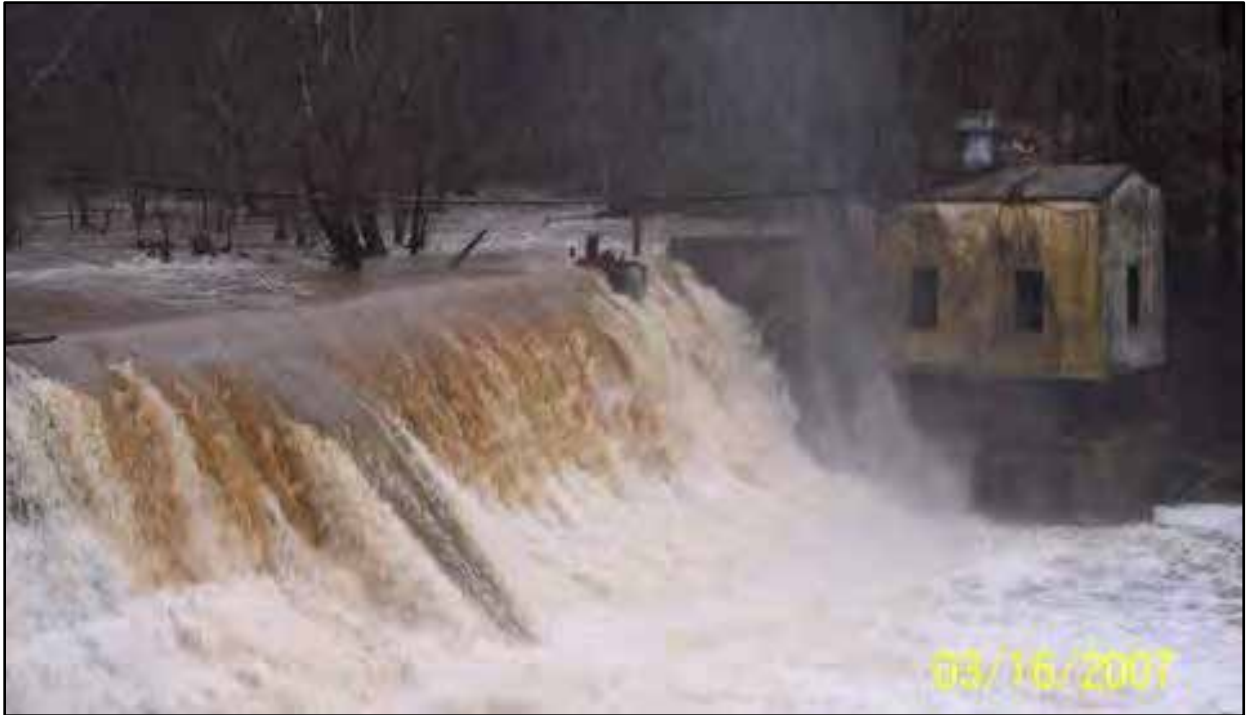
2. Power Dam during 3 inch rainfall event, view southwest (3/16/07)
