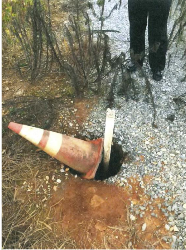
Figure 4: Shallow Monitoring Well on Phase II.
