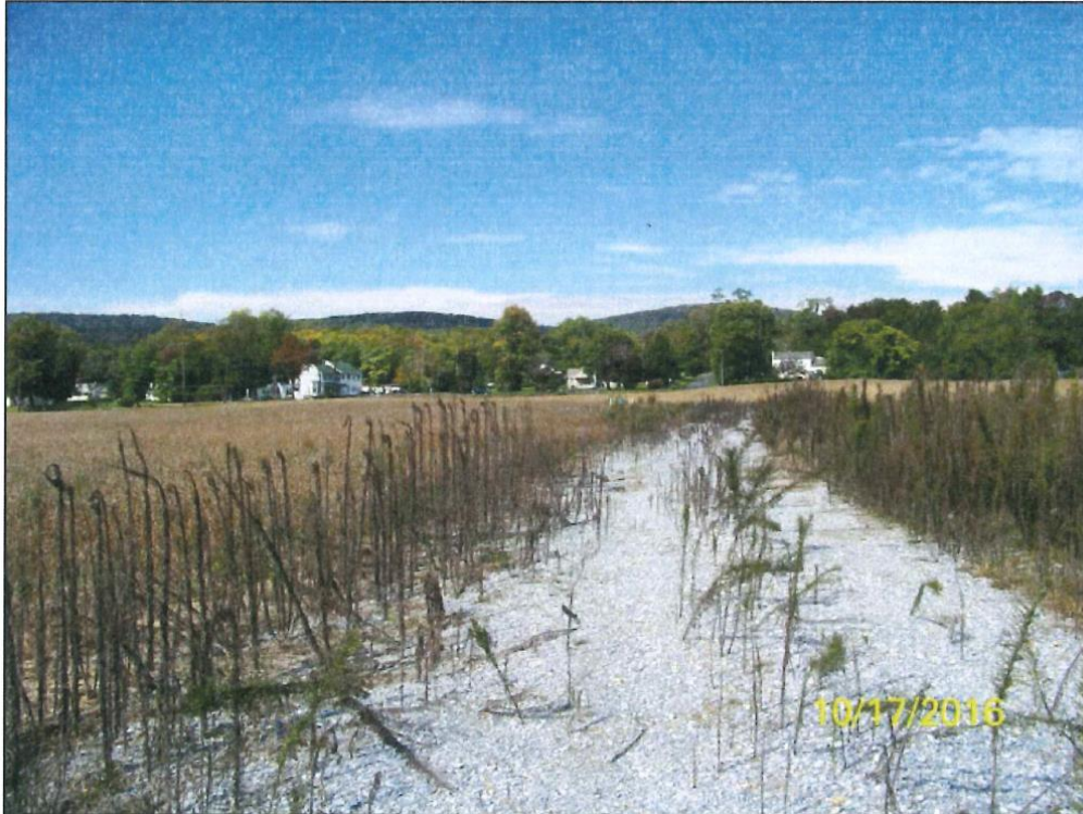
Image 8: Gravel Access Road on Phase II.
