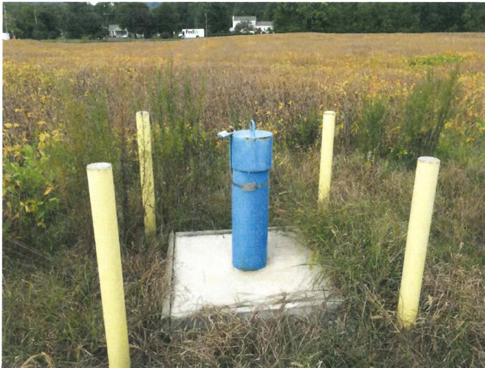
Figure 1: Deep Monitoring Well on Phase II.
